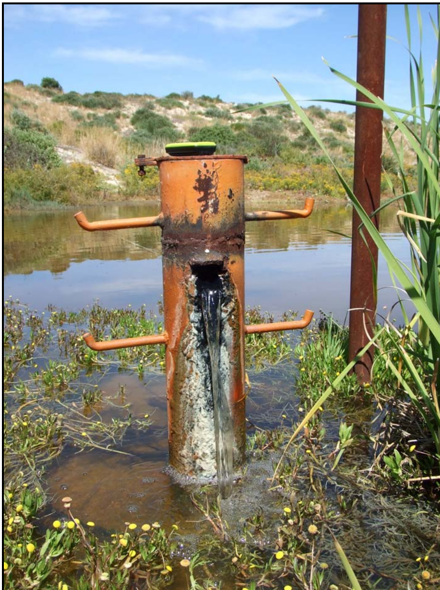
Figure 2-10 Artesian Borehole in groundwater fed pool: Evidence of 2 water tables
